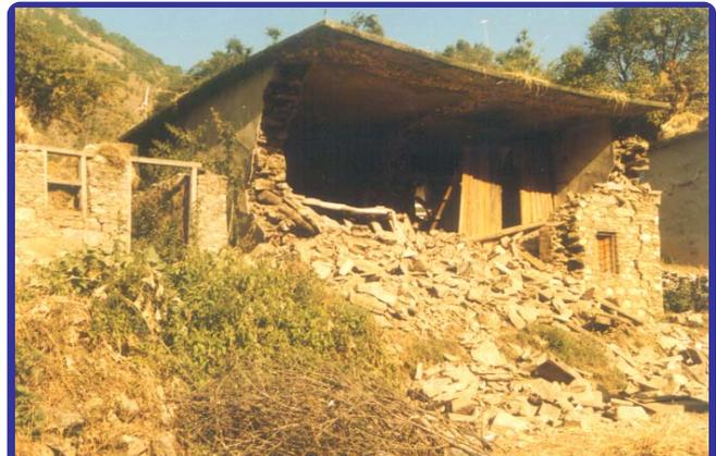
**(a) Partial collapse of stone masonry walls during 1991 Uttarkashi (India) earthquake**
